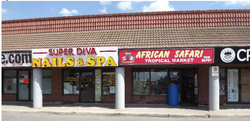
Figure 3. Ten Steeles Plaza, 1 Steeles Avenue East
