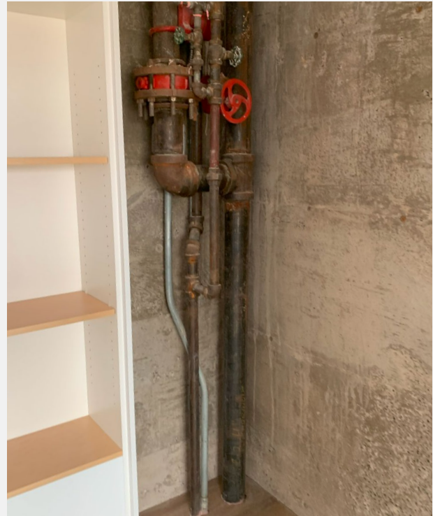
■ Figure 3. Copper piping carried over from the original structure in The Shuffle
