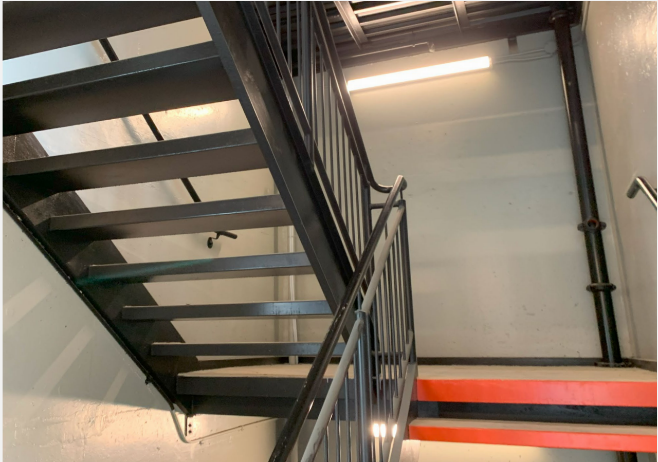
■ Figure 5. Stairwell in The Shuffle which only required minor alteration
