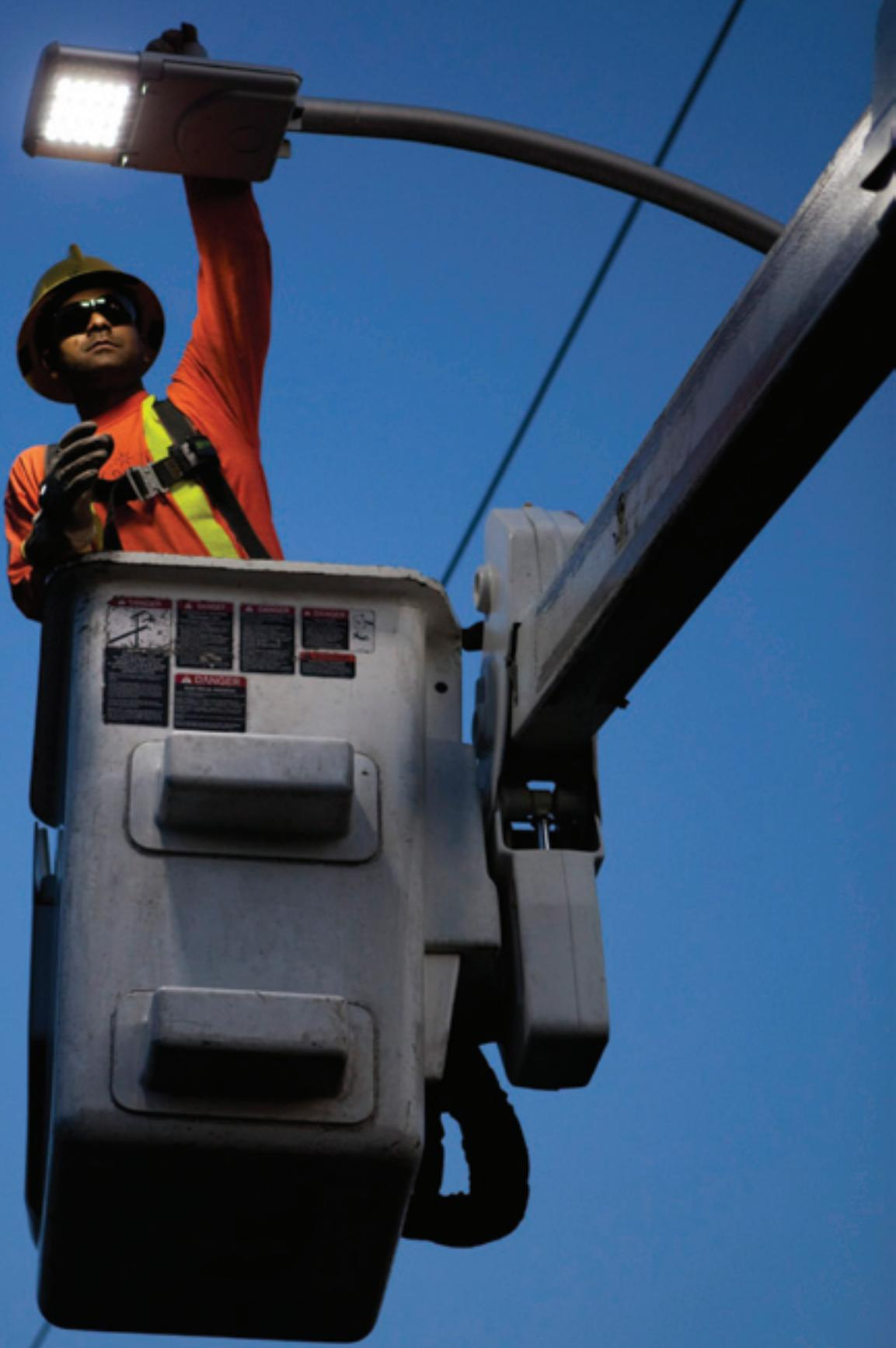
**DIRECTIONAL ILLUMINATION PERFORMANCE.** Energy savings observed in the trials tell only part of the story of LED performance. A key advantage that LED luminaires hold over conventional lamps is that the light they produce is more directional. More of the light leaving the LED luminaire reaches the pavement surface where it is needed so less – if any – light pollutes the dark sky.
